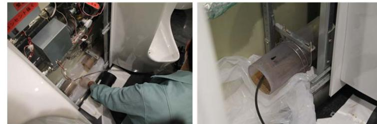
The thickness of calcified urine was estimated from the photograph of Videoscope.
